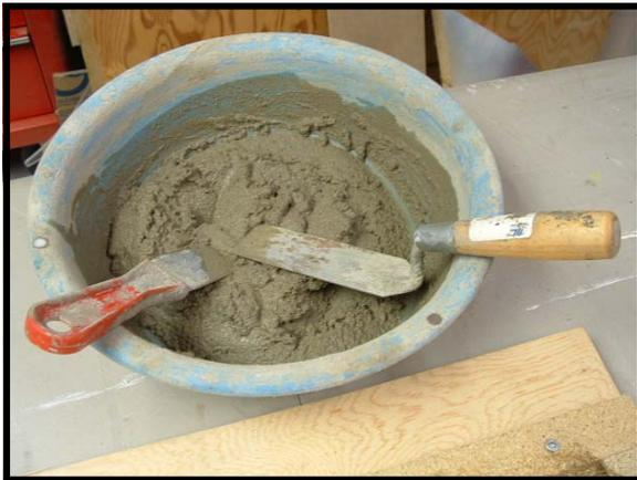
I use ordinary sand mix cement to do this. I mix it to the consistency of a thick cake batter. It must be wet enough to get in around the windows and not create air pockets. I also use “Welbond” glue in the water that I use to mix my cement. This adds a lot of strength to the cement. Proportions are about 1/2 cup mixed in a litre of water.
