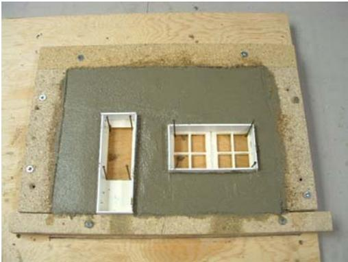
Place the second 1/4" of cement on top of the hardware cloth and when you have finished it should look like **diagram 14**
